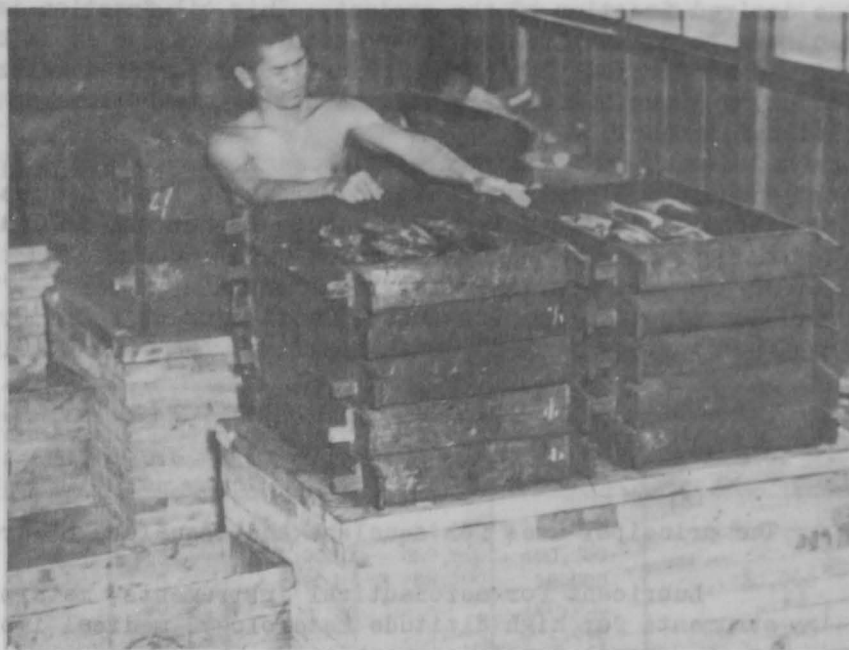
FIGURE 7 - SMOKING BOILED SKIPJACK FILLETS. FILLETS ARE PLACED IN WIRE-BOTTOMED WOODEN RACKS AND STACKED FOR SMOKING ON TOP OF BRICK FIRE-BOX.
