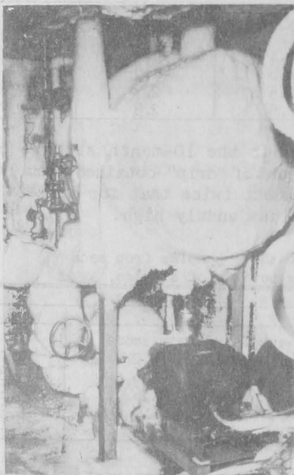
FREEZING EQUIPMENT ABOARD A MODERN TUNA CLIPPER
