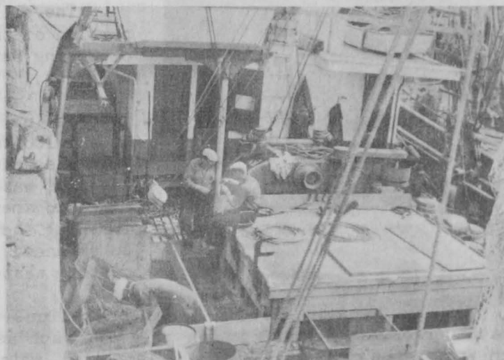
LOOKING FORWARD ON THE ALASKA; BUTCHERING TABLE IN THE FOREGROUND BEARING TWO BUTCHERING KNIVES, TRAWLING WINCH LOCATED JUST BEYOND; IN THE PORT-SIDE WALKWAY THE OPENING TO THE SHARP FREEZER CHAMBER, THE COOKING TANK, AND THE COMPARTMENT HOUSING THE STEAM GENERATOR.
