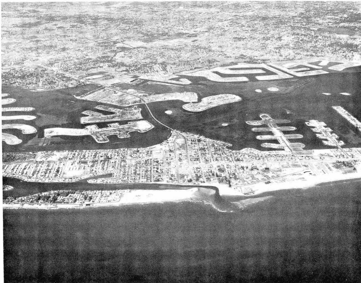
FIGURE 5.—Central Boca Ciega Bay near Corey Causeway in 1963 showing bayfill areas (photograph courtesy of Airfite, St. Petersburg, Fla.).
