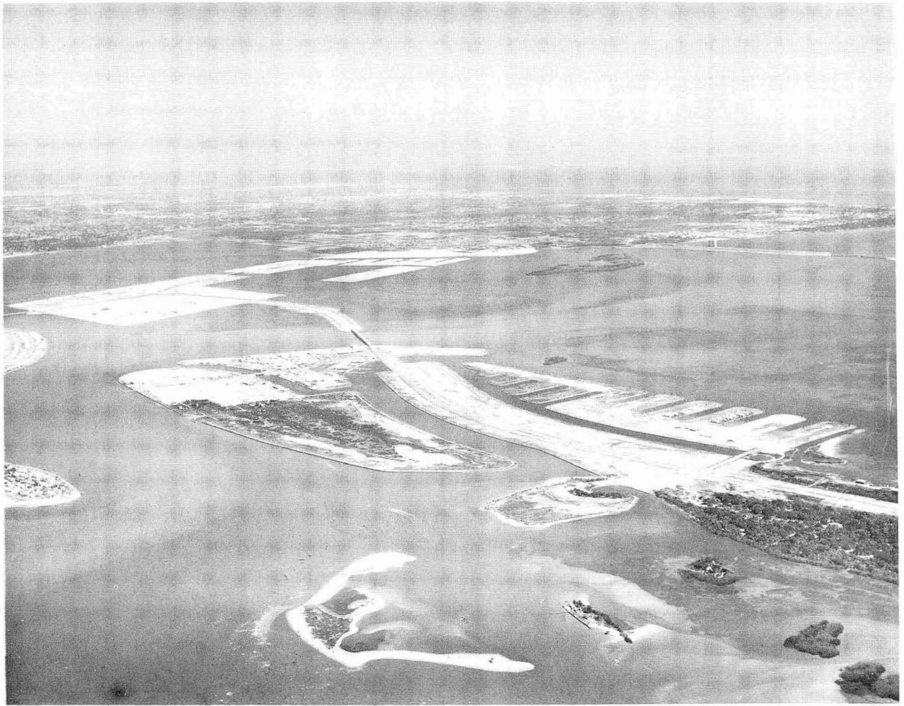
FIGURE 3.—Southern Boca Ciega Bay in 1963 showing Pinellas County Bayway and other bayfill areas (photograph courtesy of Airlite, St. Petersburg, Fla.)
