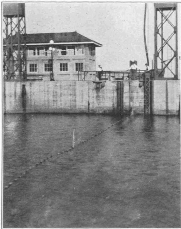
FIGURE 8.—The gate down and the corks keeping the top of the net afloat. Fish passing out of the lock, upstream, and into the lock from the lake, downstream, will be pocketed on different sides of the net
