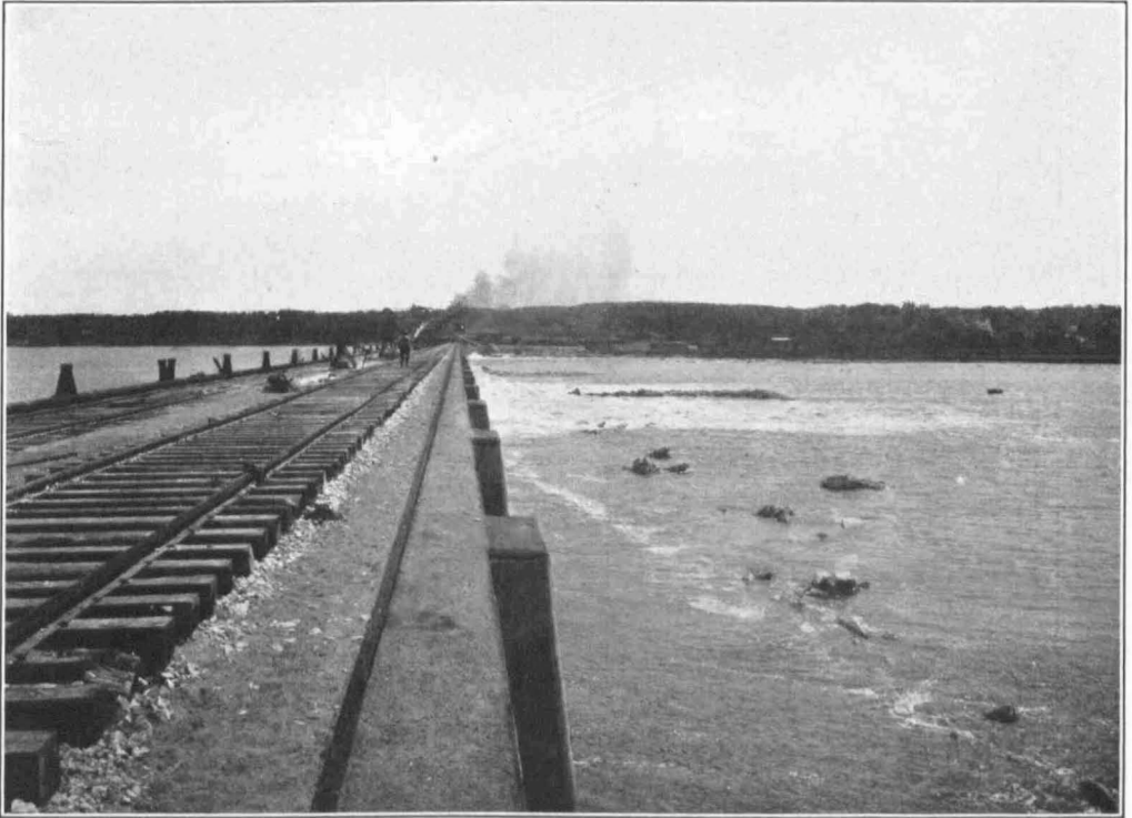
FIGURE 12.—Looking eastward over the dam in July, 1913. Exposed rocks may be seen below the spillways. (This photograph was taken soon after the dam was completed)
