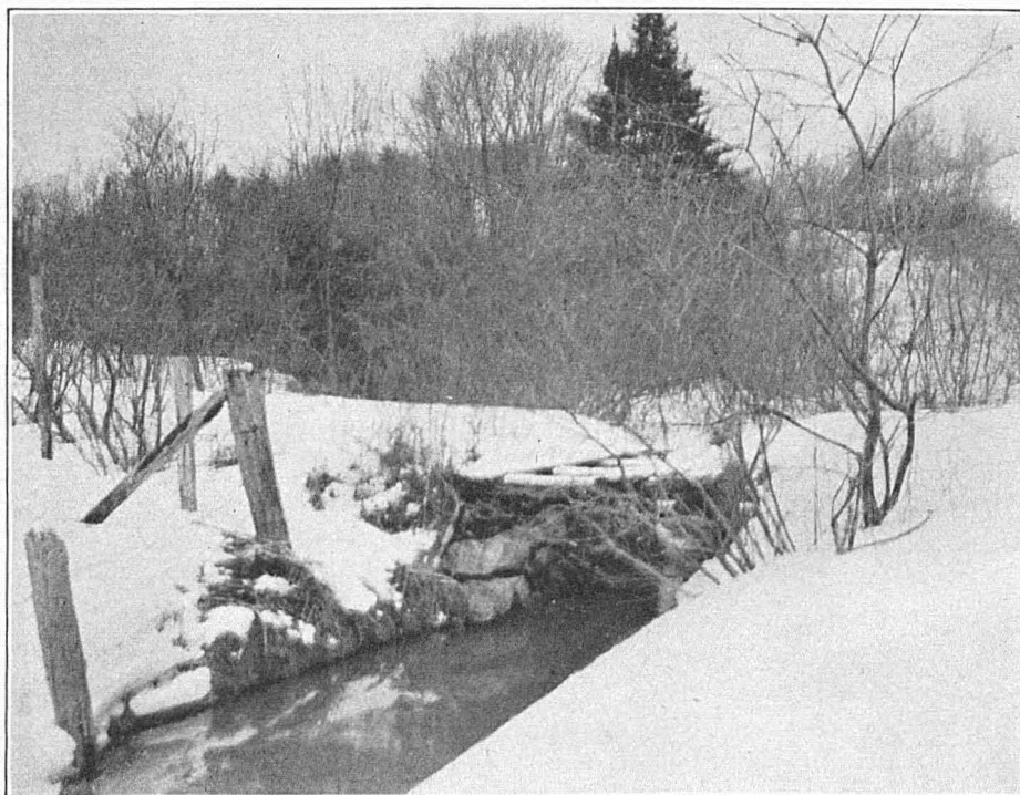
FIG. 5.—Porters Landing smelt brook just below the remains of the bridge shown in Figure 4. Extremely high tides reach this point. Taken in the early spring about 2½ weeks before breaking up of ice
