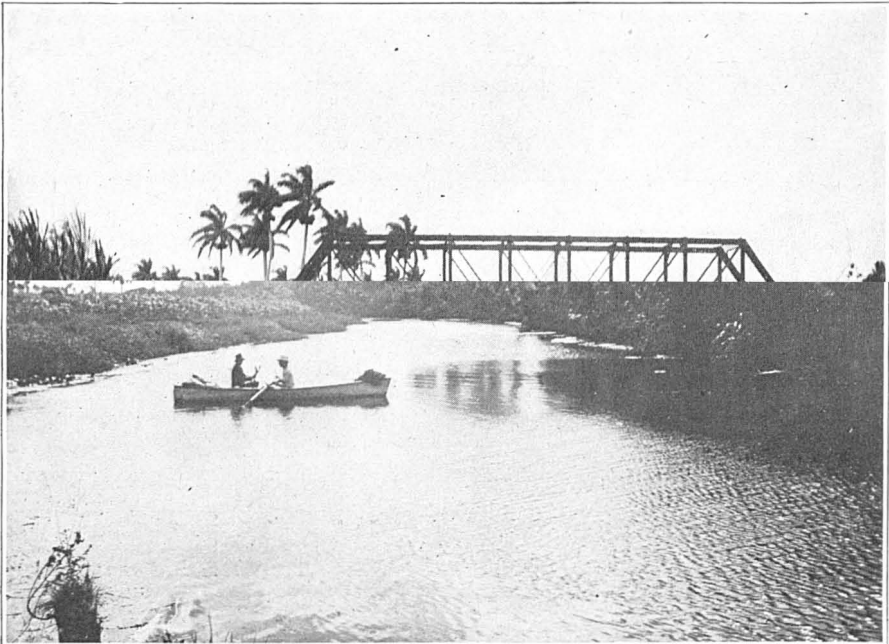
SAN JUAN RIVER, LOOKING UPSTREAM FROM THE FIRST BEND ABOVE THE UNITED HABANA RAILROAD BRIDGE.
