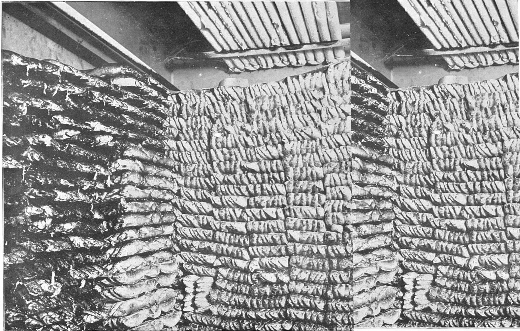
STORAGE ROOM OF AMMONIA REFRIGERATING PLANT AT CINCINNATI, CONTAINING LAKESIDE STORAGE ROOM OF AMMONIA REFRIGERATING PLANT AT CINCINNATI
