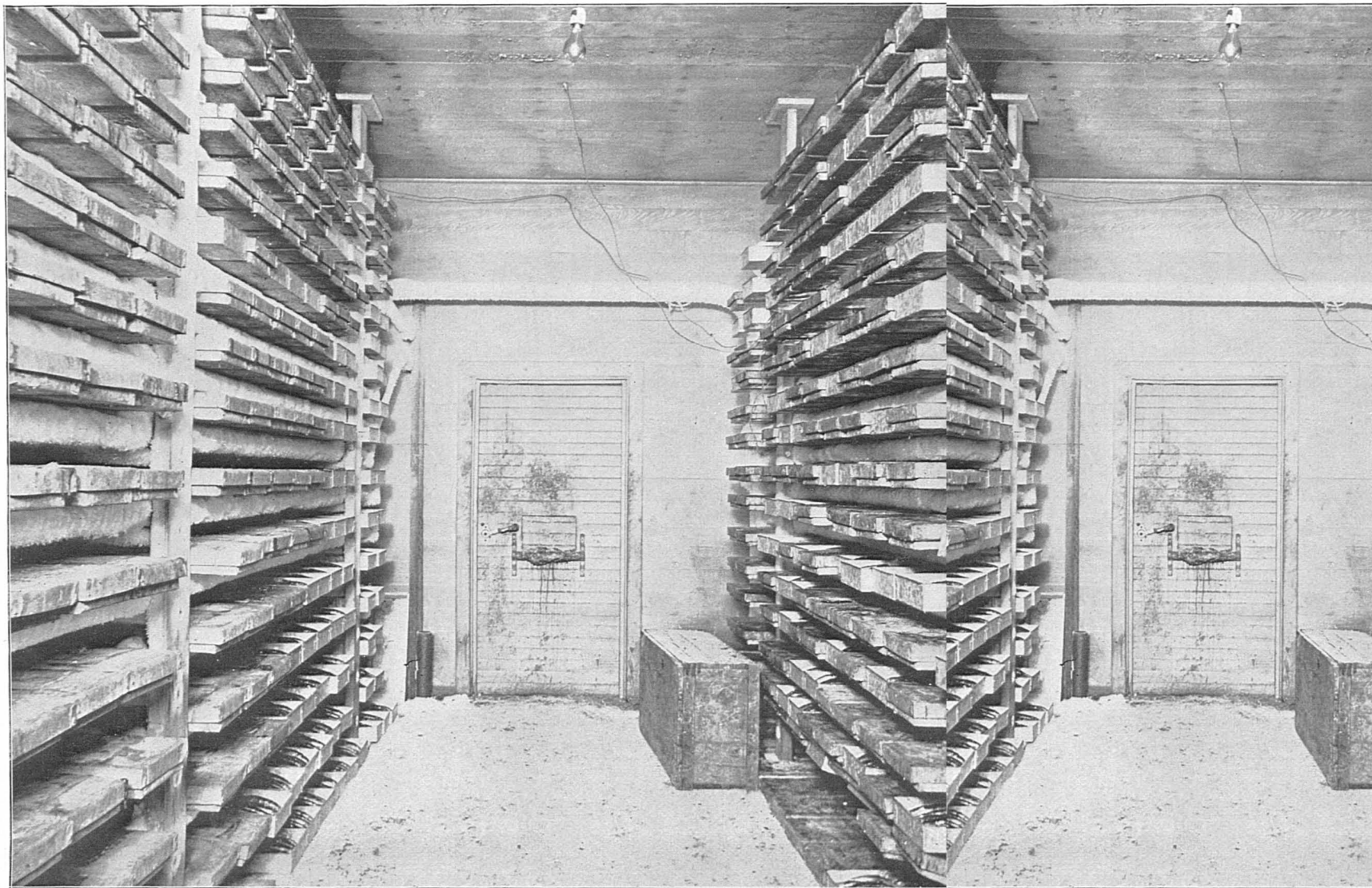
FREEZING ROOM OF AMMONIA PLANT AT CINCINNATI, OHIO (CINCINNATI FISH AND OYSTER COMPANY), SHOWING COILS OF CIRCULAT CINCINNATI, OHIO (CINCINNATI FISH AND OYSTER COMPANY)
