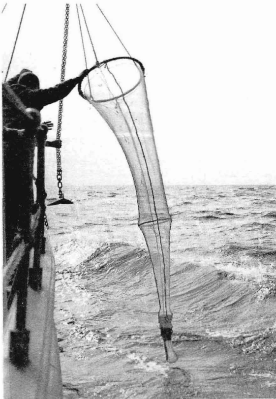
FIGURE 4.—Views of the high-speed net, showing attachment of towing bridles and depressor.
