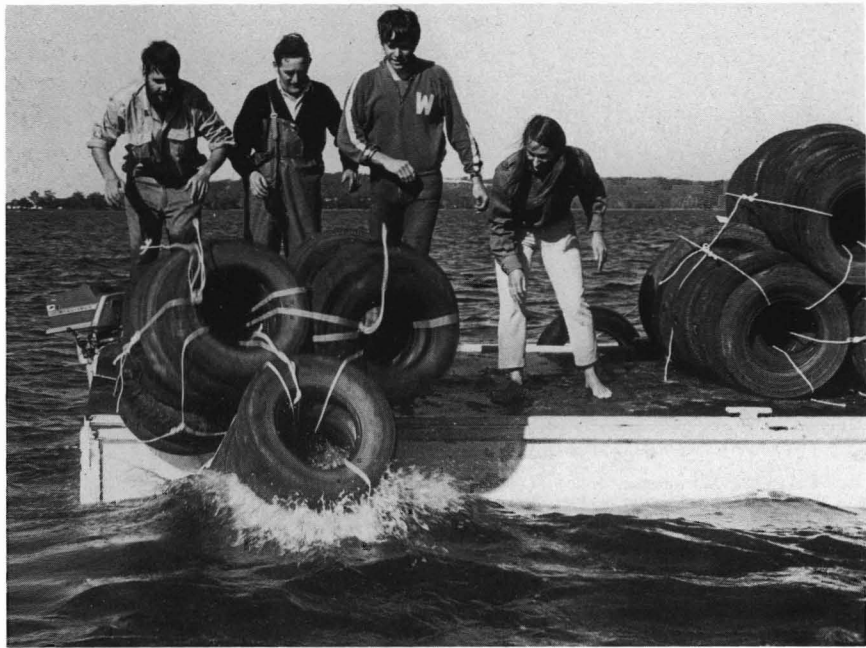
Figure 2.—Tire reef units being laid in Lake Macquarie, 1970.
