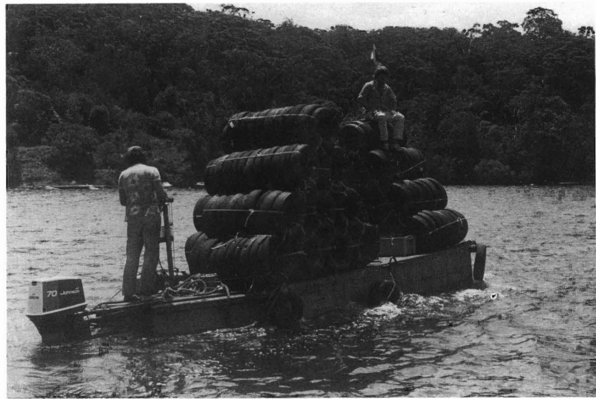
Figure 6.—Tire units being barged to Port Hacking artificial reef site, 1977.
