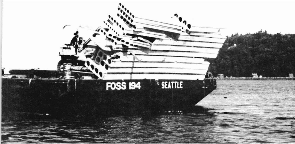
Figure 4.—Scrap concrete used for habitat enhancement construction.
