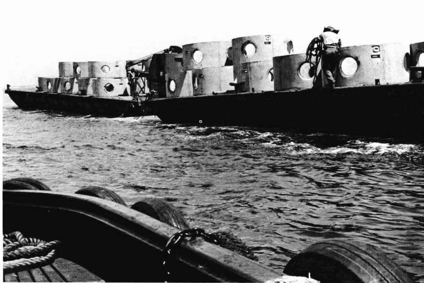
Figure 3.—Concrete units adapted from Japanese-style units prior to placement off Long Island, N.Y., during 1964-65. (Photo courtesy of the New York State Department of Environmental Conservation.)
