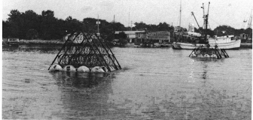
Figure 16.—Reef units being towed to site off Jacksonville, Fla.
