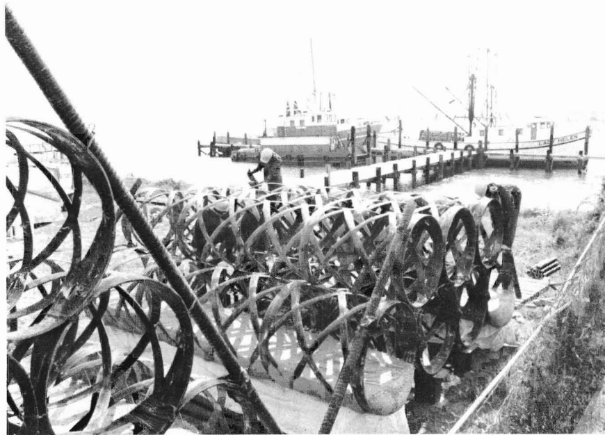
Figure 14.—Workers fibreglassing all connecting points.
