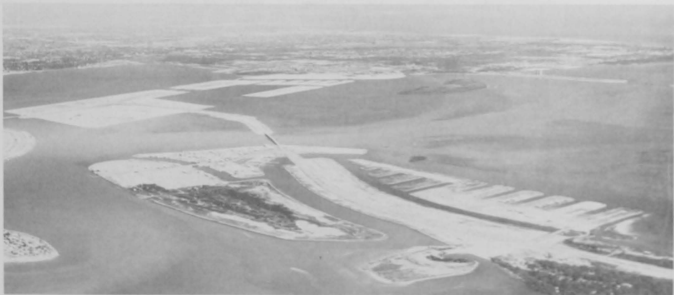
Completed dredge and fill project for housing development.
