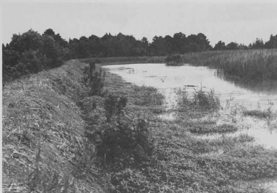
Example of marsh impoundment—prevents tidal exchange, thus nutrient exchange and the ingress and egress of estuarine-dependent organisms.
