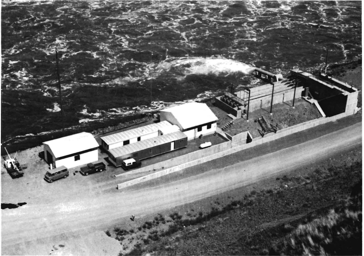
Figure 6.—Overall view of fish holding and marking facility at Lower Granite Dam (shown from left to right are: shop, laboratory and office buildings, marking facility, fish holding facility, and upwell and grader units).
