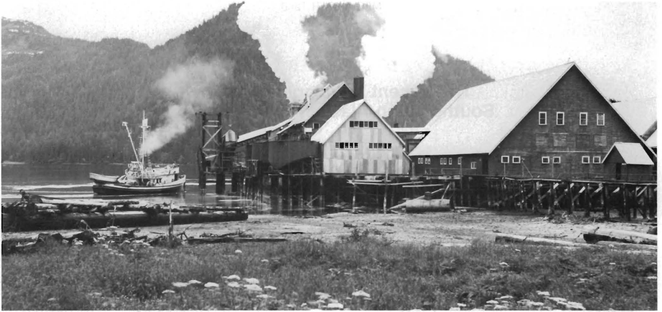
Herring reduction plant, Big Port Walter, Alaska, with seiners both approaching and leaving the unloading dock. The entire operation was dependent on highly efficient Pelton wheel power. Circa 1930.
