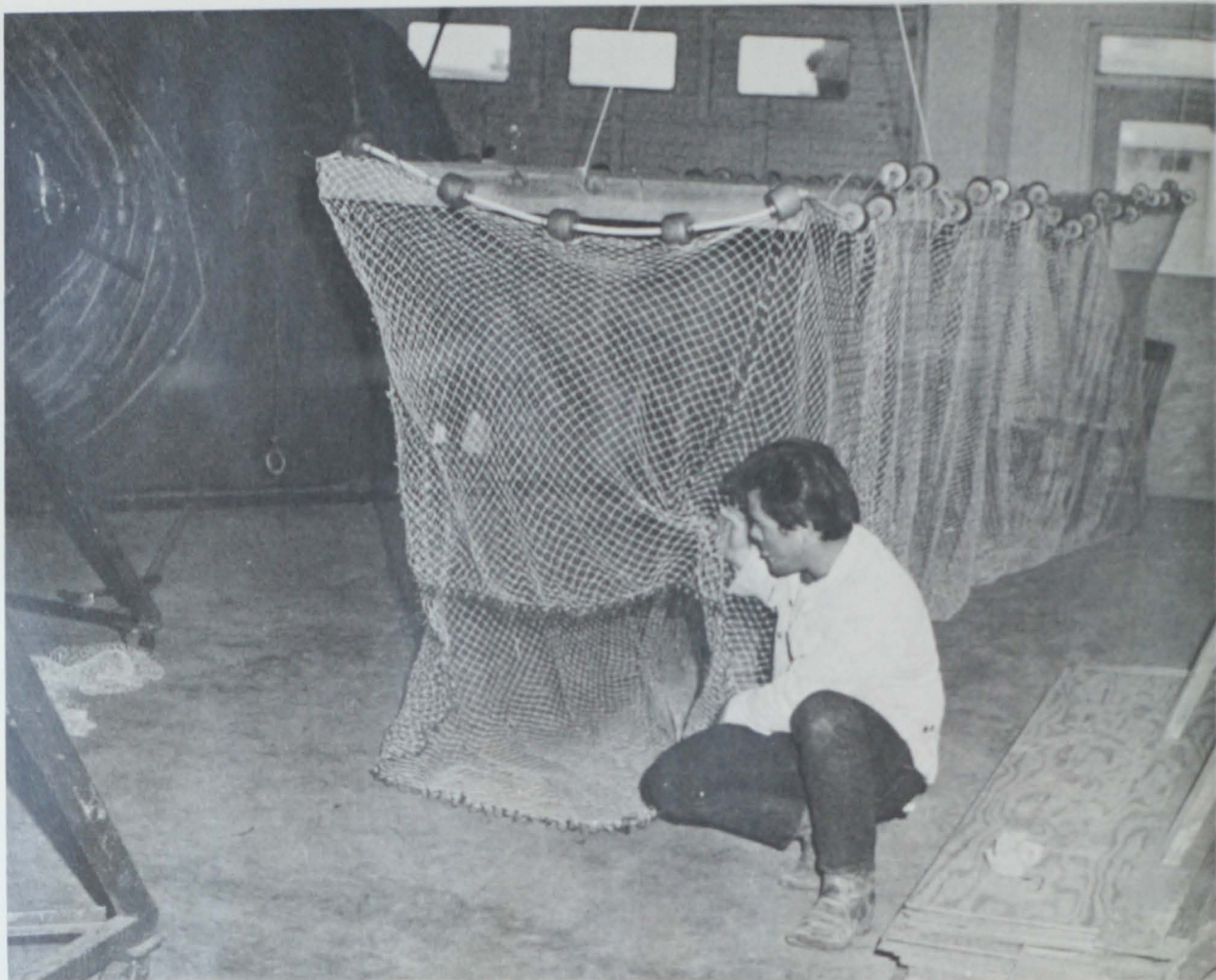
Fig. 7 - Live car in final stages of construction showing 2 by 4-foot-wide opening left for coupling ring.
