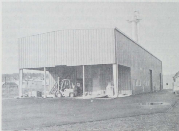
Fig. 8 - The solvent is recovered by distillation in 54-foot tower that extends above roof line of plant.
