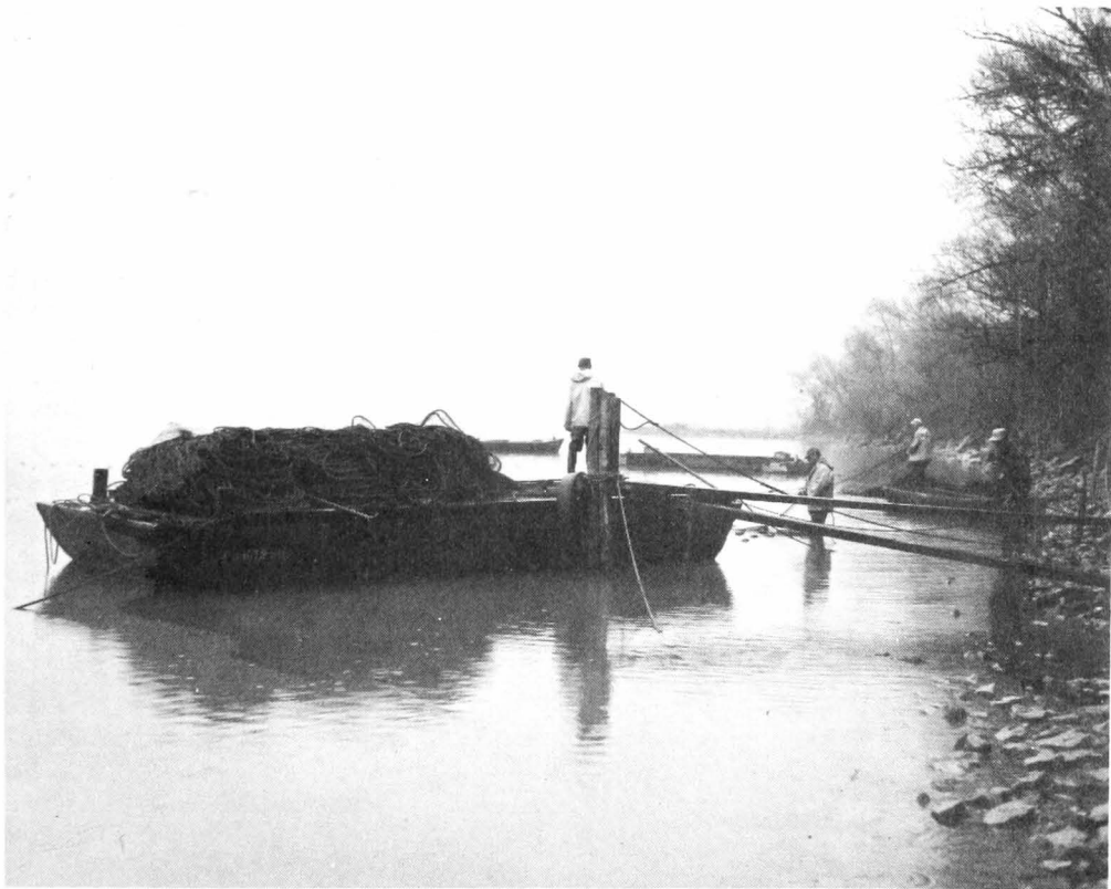
Figure 5.--Seine barge, measuring 20 by 8 feet, used in the haul seine fishery.
