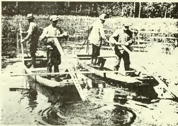
Fig. 46. The Mowing of water plants with the Drailich reed scythe. The lever arms, on whose ends are the half-moon shaped scythe blades, are moved from side to side in unison.
