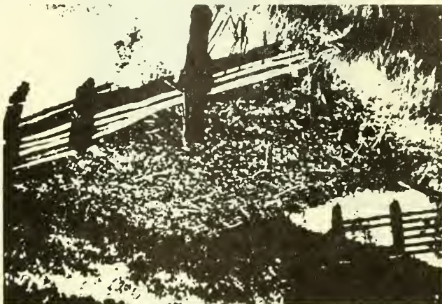
Fig. 8. A simple filter erected in the water inlet for the detention of fishes and fish brood and for superficial water cleansing.
