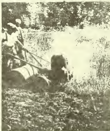
Fig. 51. Siemens small pulverizer in the cultivation of a weakly reeded brood pond. Front, the well pulverized and thoroughly mixed pond bottom in one work round.
