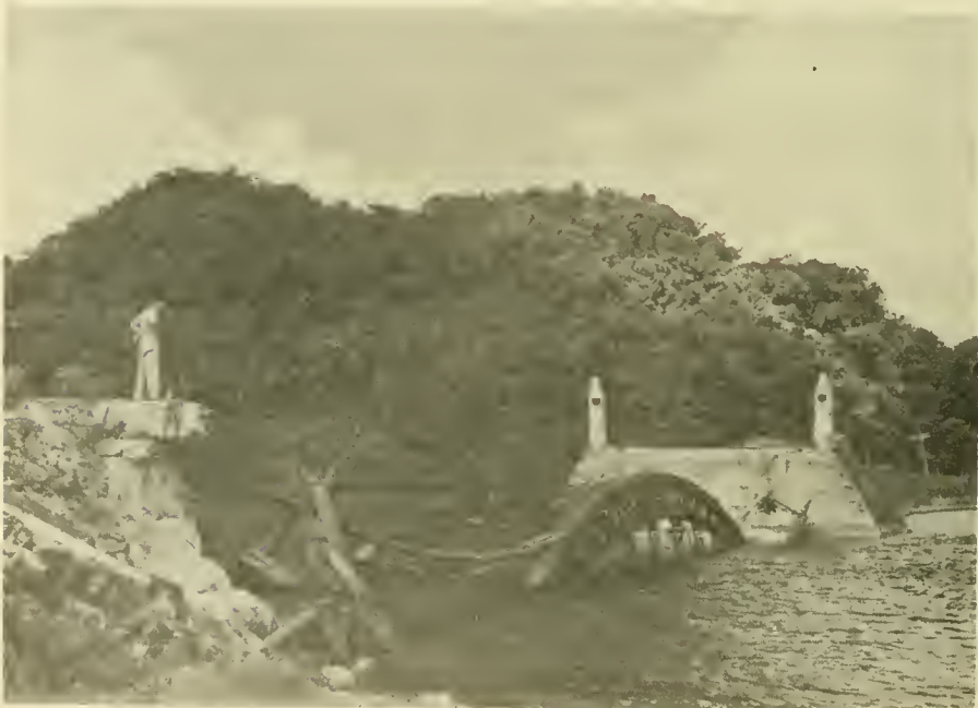
Figure 23... Palau -- Koror. Bombed bridge blocking navigation. July 1946
