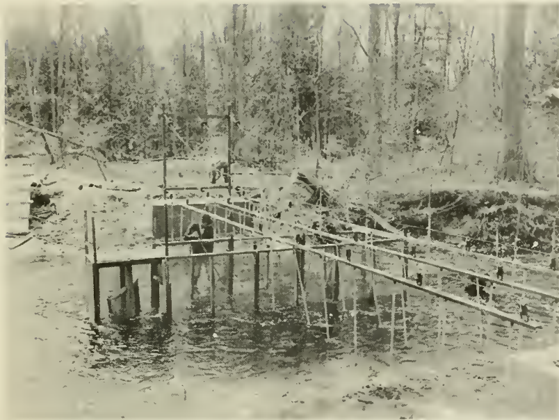
Figure 8. Electromechanical weir and trap installed in Squaw Creek in 1952.
