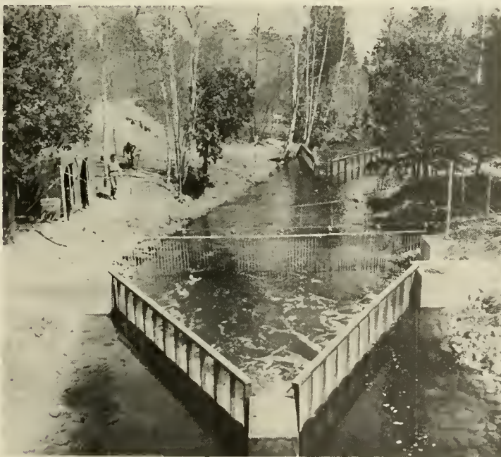
Figure 10. Electrical barrier installed in Carp Creek in 1952 with upper and lower checking weirs.
