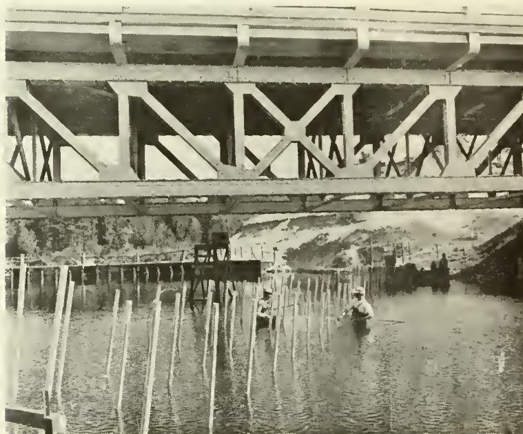
Figure 1. Experimental electromechanical weir and trap installed in the Ocqueoc River in 1951.
