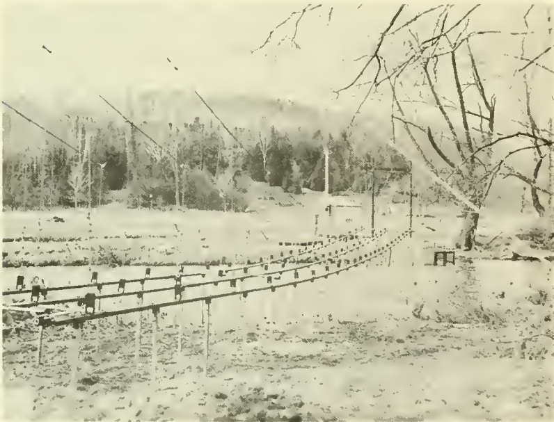
Figure 5. Electromechanical weir and trap installed in the Kewaunee River in 1952.
