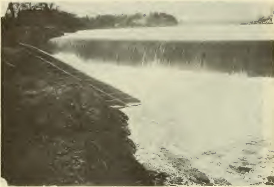
Figure 6.-- General View of Lawrence Fishway Tailwater Elevation 17 ft. (above mean sea level) Note extreme turbulence. Shad do not approach the fishway under these water conditions.
