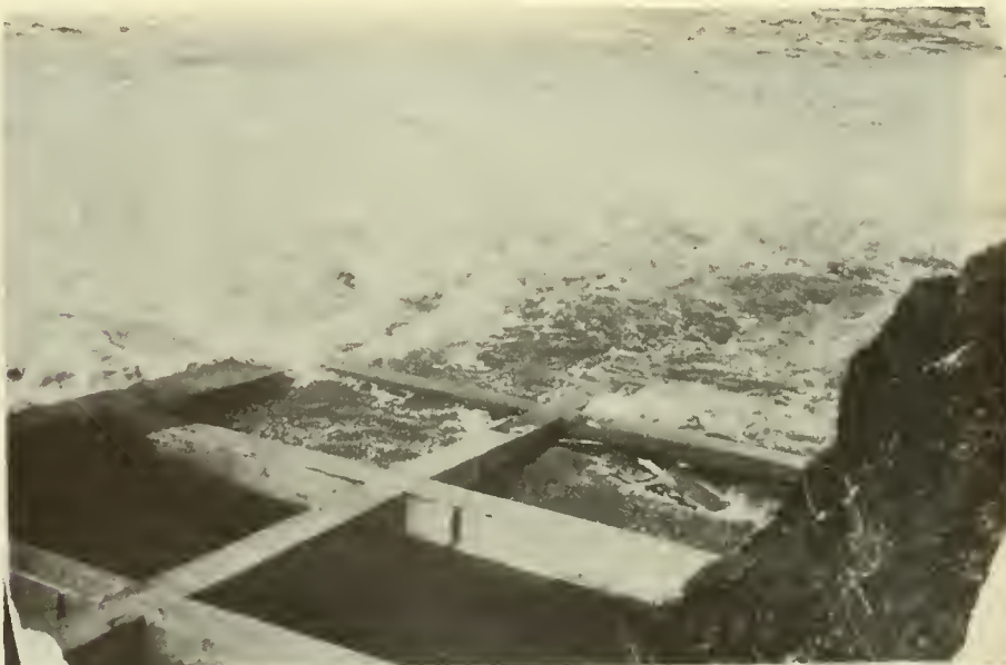
Figure 7.-- Flooded Fishway Entrance Tailwater Elevation 17 ft. (above mean sea level).
