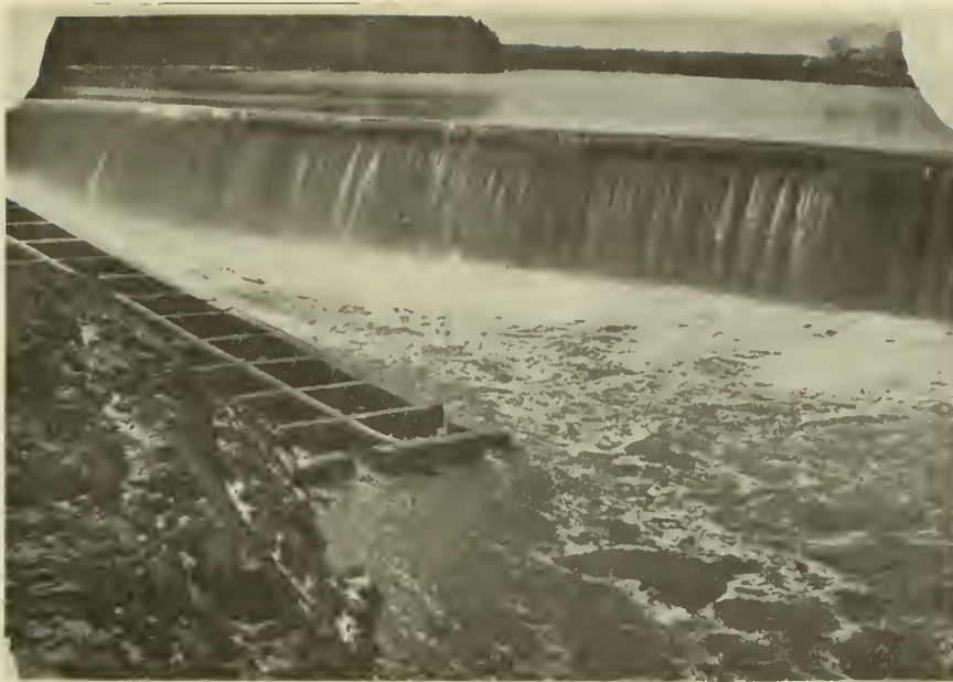
Figure 4.-- General View of Lawrence Fishway
