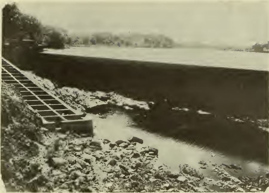
Figure 8.-- General View of Lawrence Fishway Tailwater Elevation 7 ft. (above mean sea level) No water over spillway. Shad are unable to reach the fishway under these conditions.
