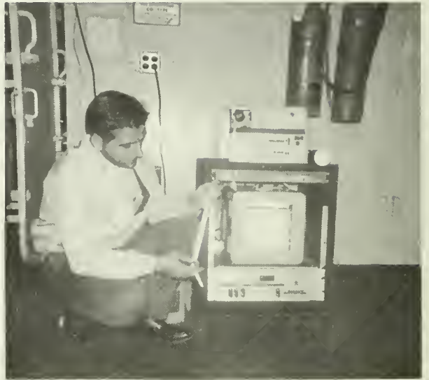
Figure 2.--Reading the paper tape punched by the reperforator on top of the electronic rack which holds the recorder and digitizer encoder unit.
