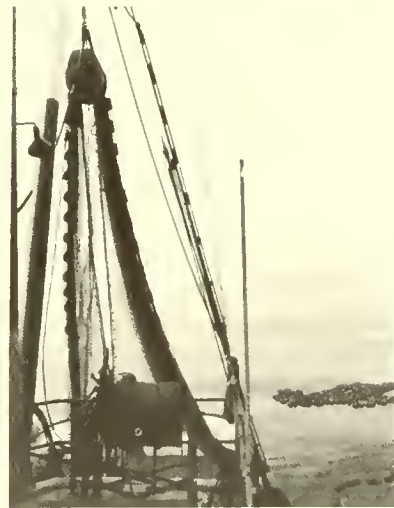
⑧ Net being pulled aboard seiner by power block
