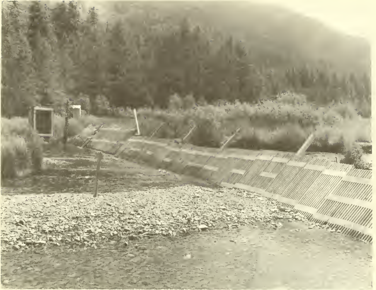
Figure 9.--Weir site at West Fork, Oisen Creek.
