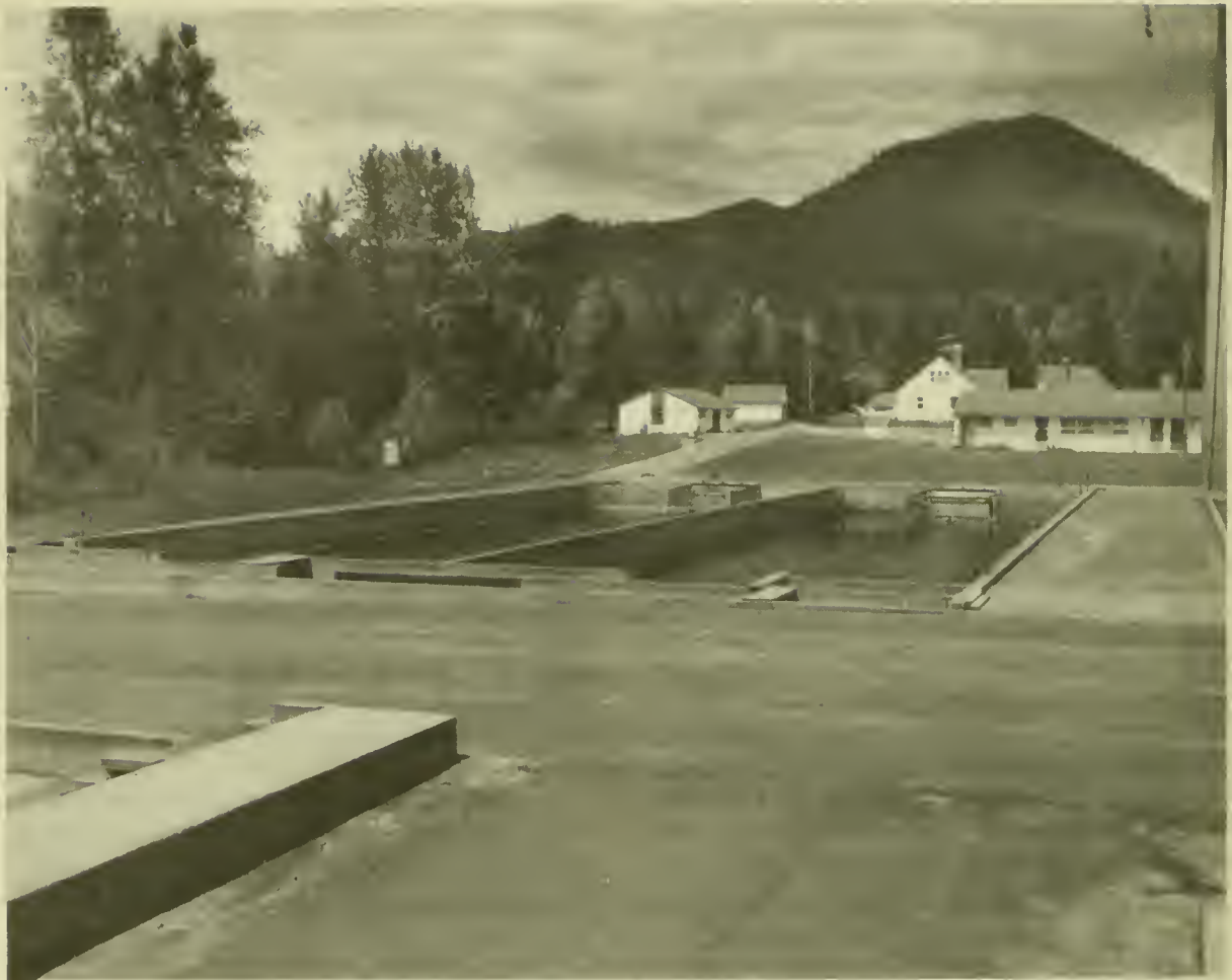
Figure 4.--Concrete holding pond for adult salmon, Carson National Fish Hatchery.
