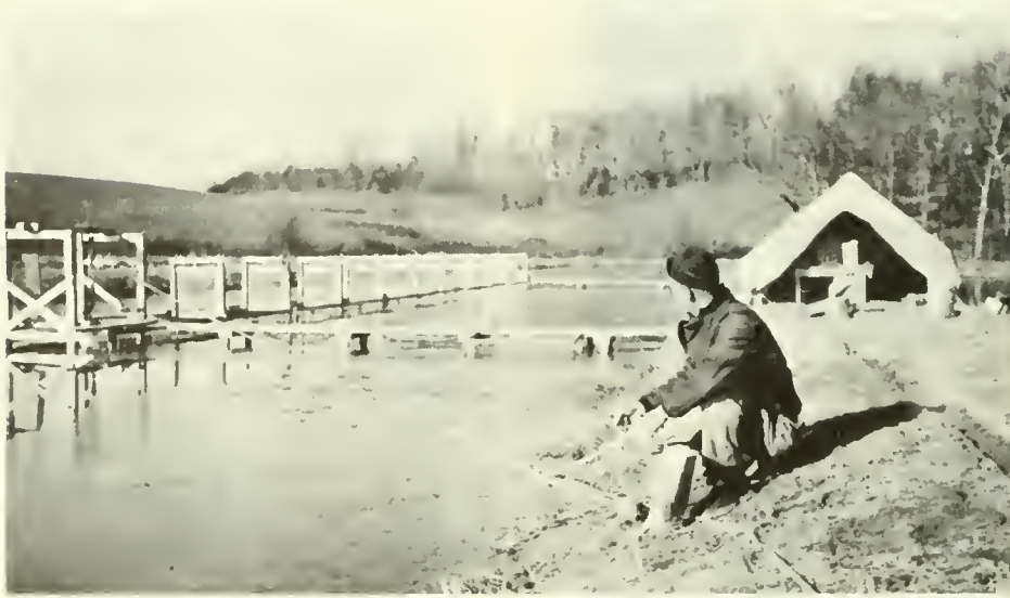
Figure 4.--Gates being held up as during a sound or a control run.
