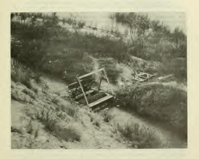
Figure 7.-- A rotary drum screen in a diversion ditch on the Wenatchee River. A by-pass provides passage for the fingerlings from in front of the drum screen back to the river.
