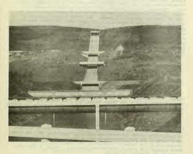
Figure 4.-- Irrigation ditches from the Yakima River crossing the Terrace Heights Wasteway of the Roza Canal near Yakima, Washington. Crossing from top to bottom are: Roza Canal; Selah - Moxee Canal; Highway bridge; Ray Slavin Branch of the Moxee Ditch; Middy Branch of the Moxee Ditch; Union Gap Ditch.
