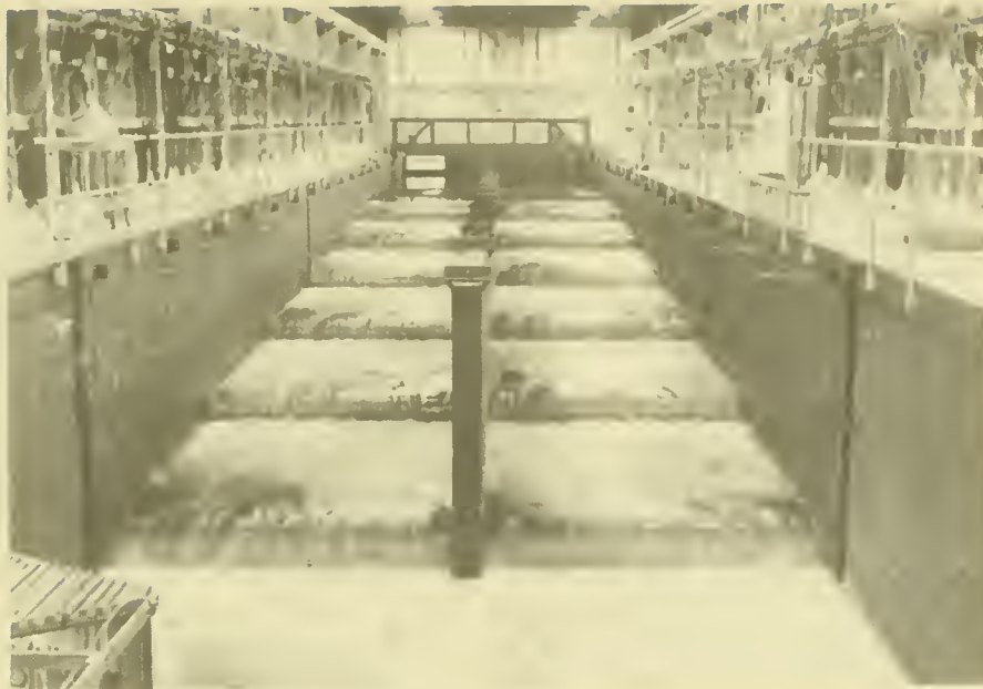
Figure 4.--The two 1:16-slope fishways in the experimental flume.
