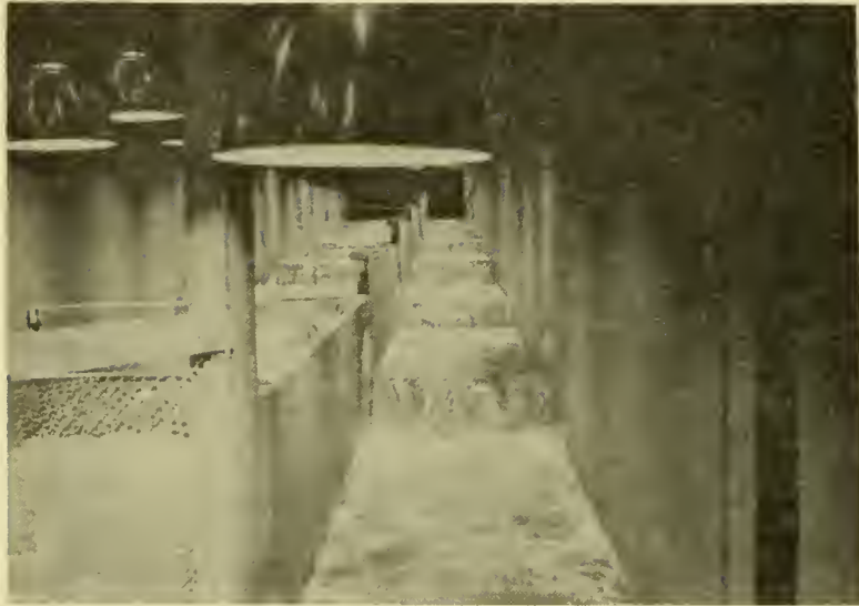
Figure 1. --Looking upstream on test fishway (on right). Mesh barrier in foreground prevented fish from entering section of fishway to the left of partition wall.
