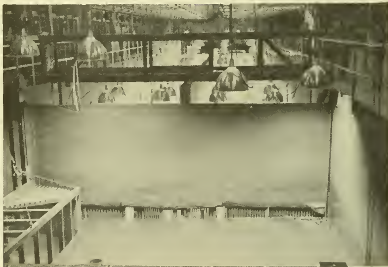
Figure 4.--View of collection pool (foreground). Barrier extends 8 feet above water surface to prevent fish from jumping into fishway area upstream of pool.
