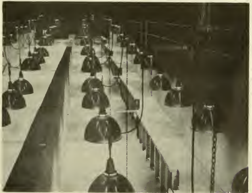
Figure 4.--The lighted fishway. Upper five pools of fishway are shown on extreme right.
