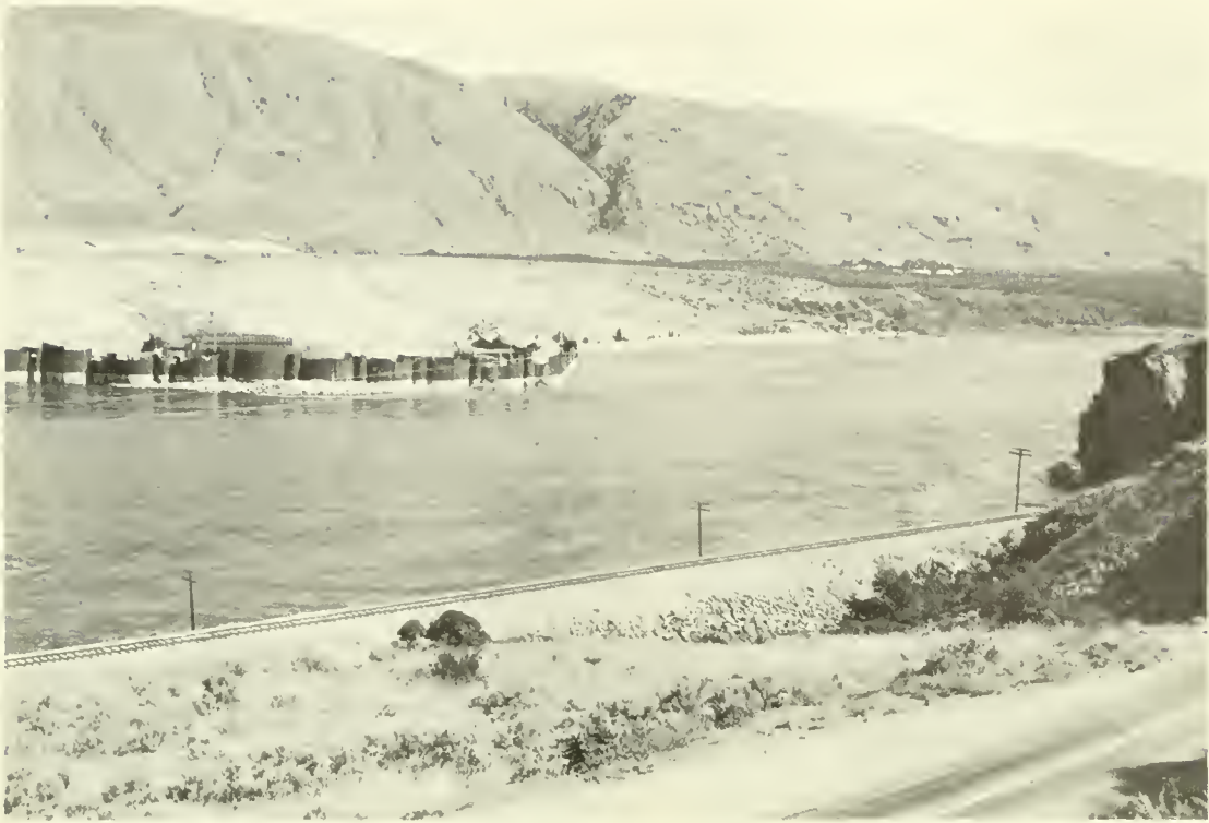
Rocky Reach Dam Construction
