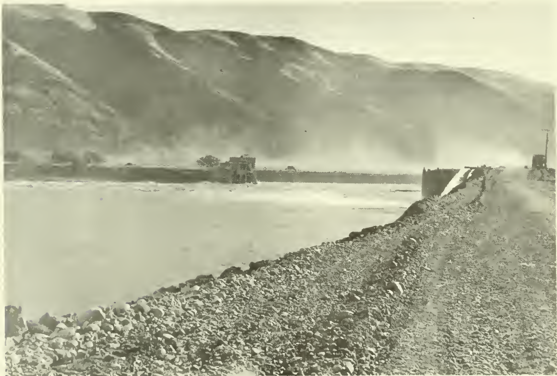
Priest Rapids Dam Construction
