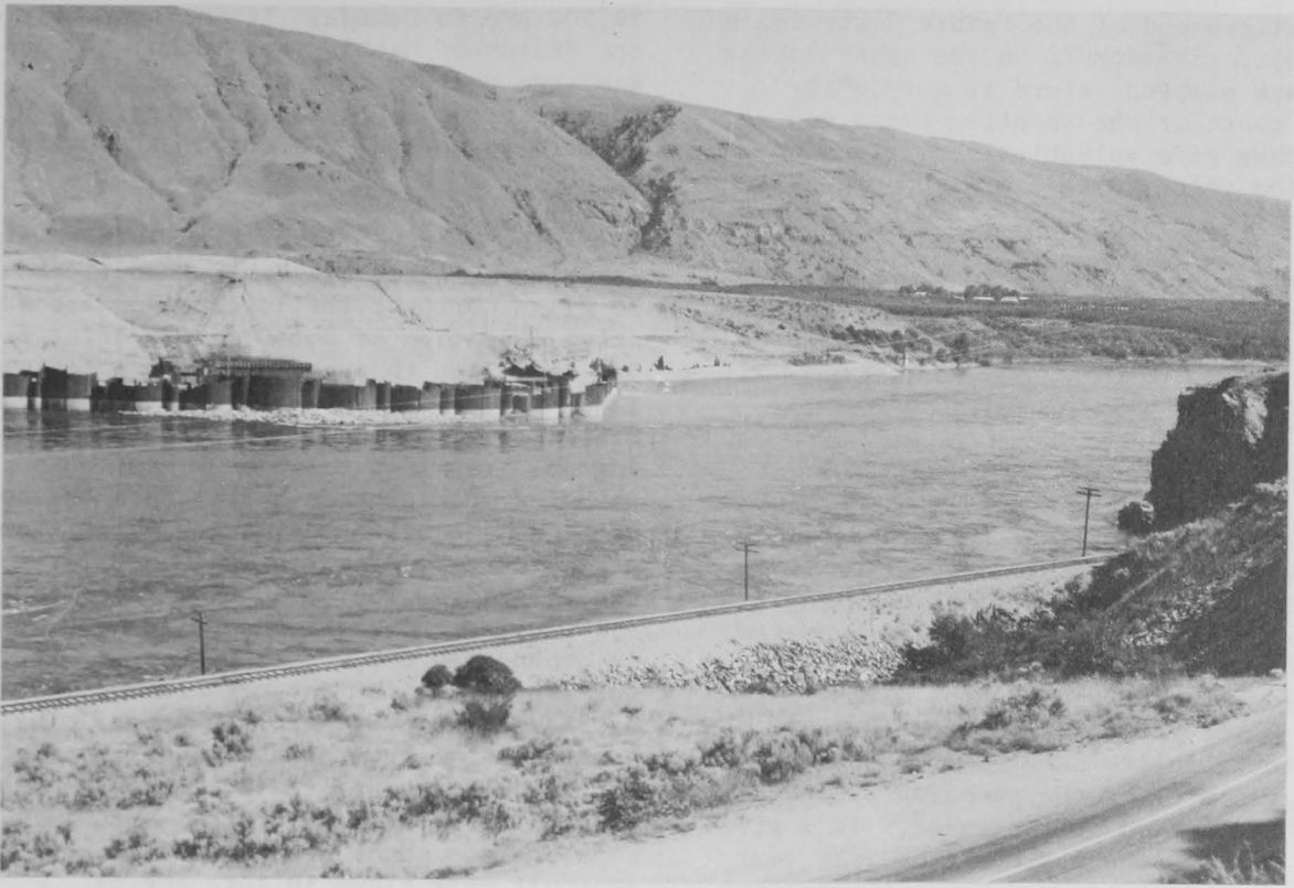
Rocky Reach Dam Construction
