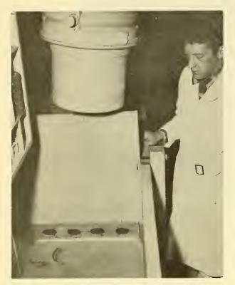
Figure 9.--An experimental tank, located along one of the walkways, equipped to evaluate small tunnels to be used in passing downstream migrating fingerlings. Infrared lamp hanging above tank.
