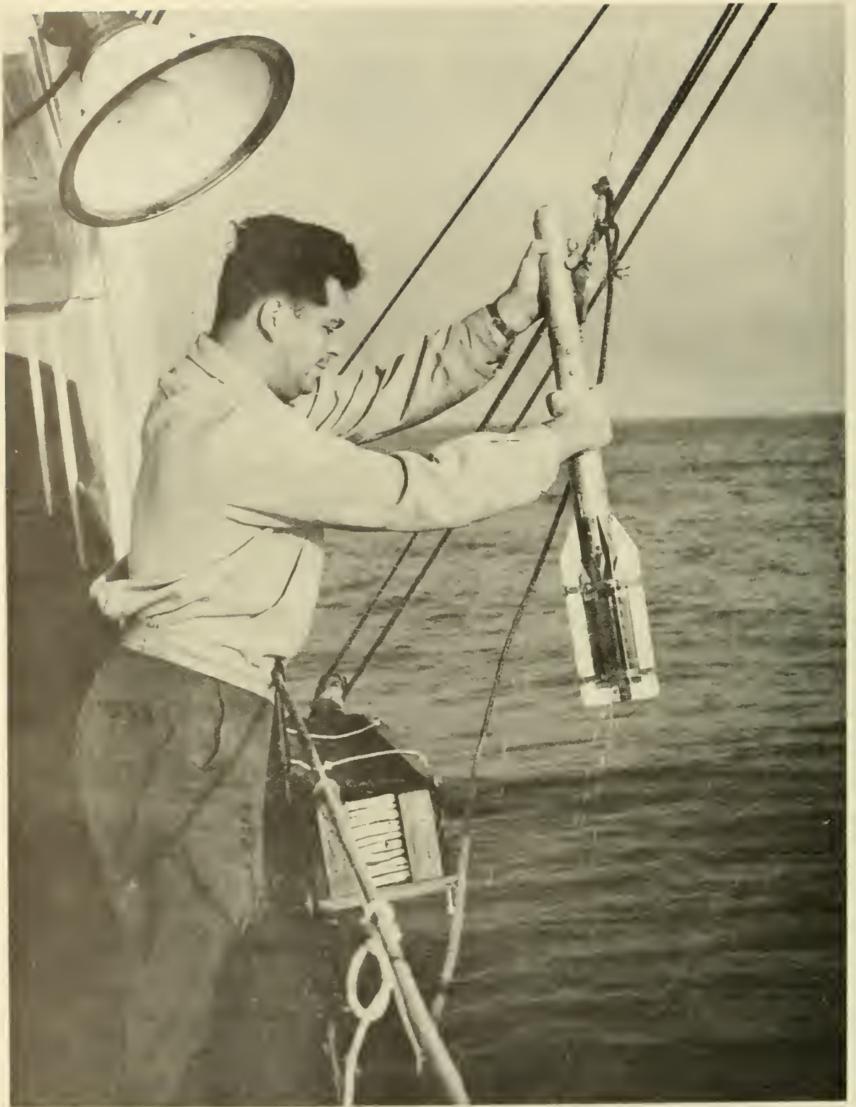
Figure 4.--Retrieving bathythermograph at end of cast.
