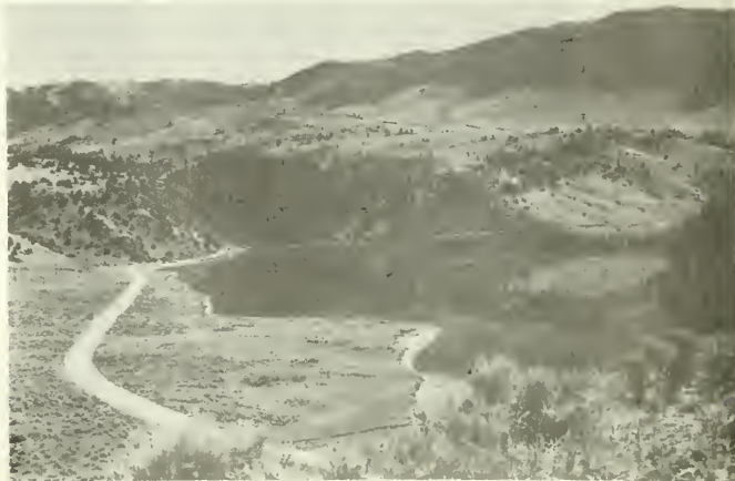
Fig. 4. Lower portion of Madison Reservoir. Madison Dam is located about 1-1/2 miles down Bear Trap Canyon, the head of which is evident in the background. (Photo by L. E. Hiner).
