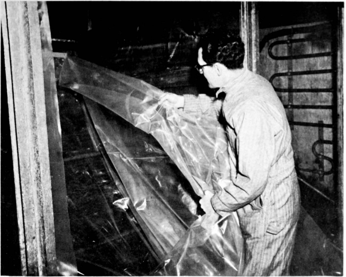
Figure 1.—Removal of disposable plastic sheeting. The surfaces behind the sheeting are clean and dry.
