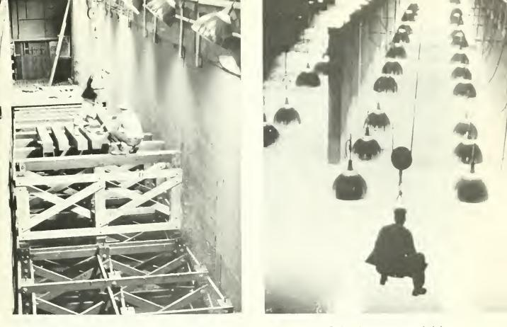
Figure 5.—Experimental fishways under construction. Careful planning and great ingenuity are required in building temporary structures capable of supporting and controlling large volumes of water. Figure 6.—Full-scale experimental fishways in operation. Standard lighting conditions are created by mercury-vapor lamps. Picketed barriers and release gates for the control of fish have yet to be erected.
