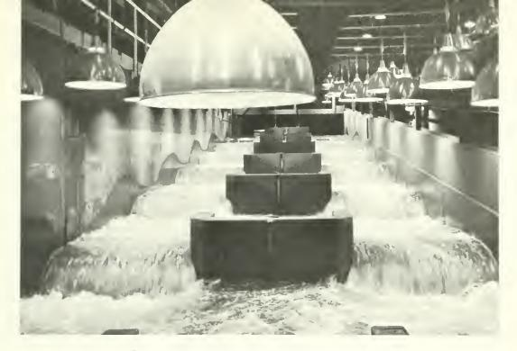
Figure 23.—Ice Harbor design fishway in operation.
