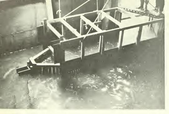
Figure 3.—Entrance to the fish collection pool. Fish swim into the laboratory through a narrowing funnel that prevents them from leaving.
