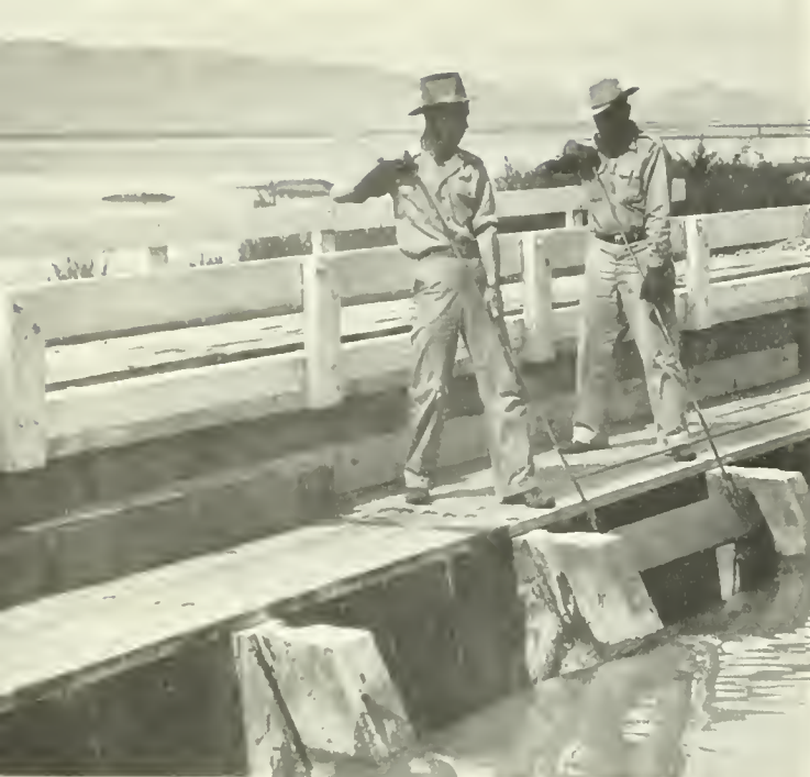
Water-control gate at Bear River Refuge.
