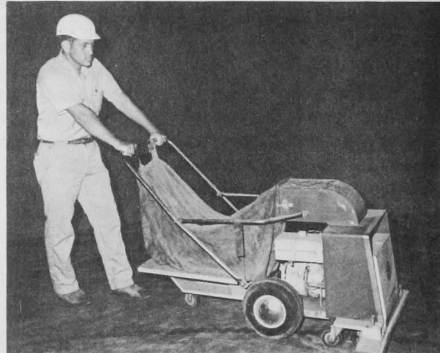
Figure 5. Use of vacuum machine aids in dust control.
