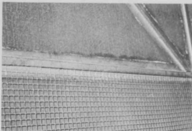
Figure 2. Dual type screening: insect screen covered with “rat wire.”
