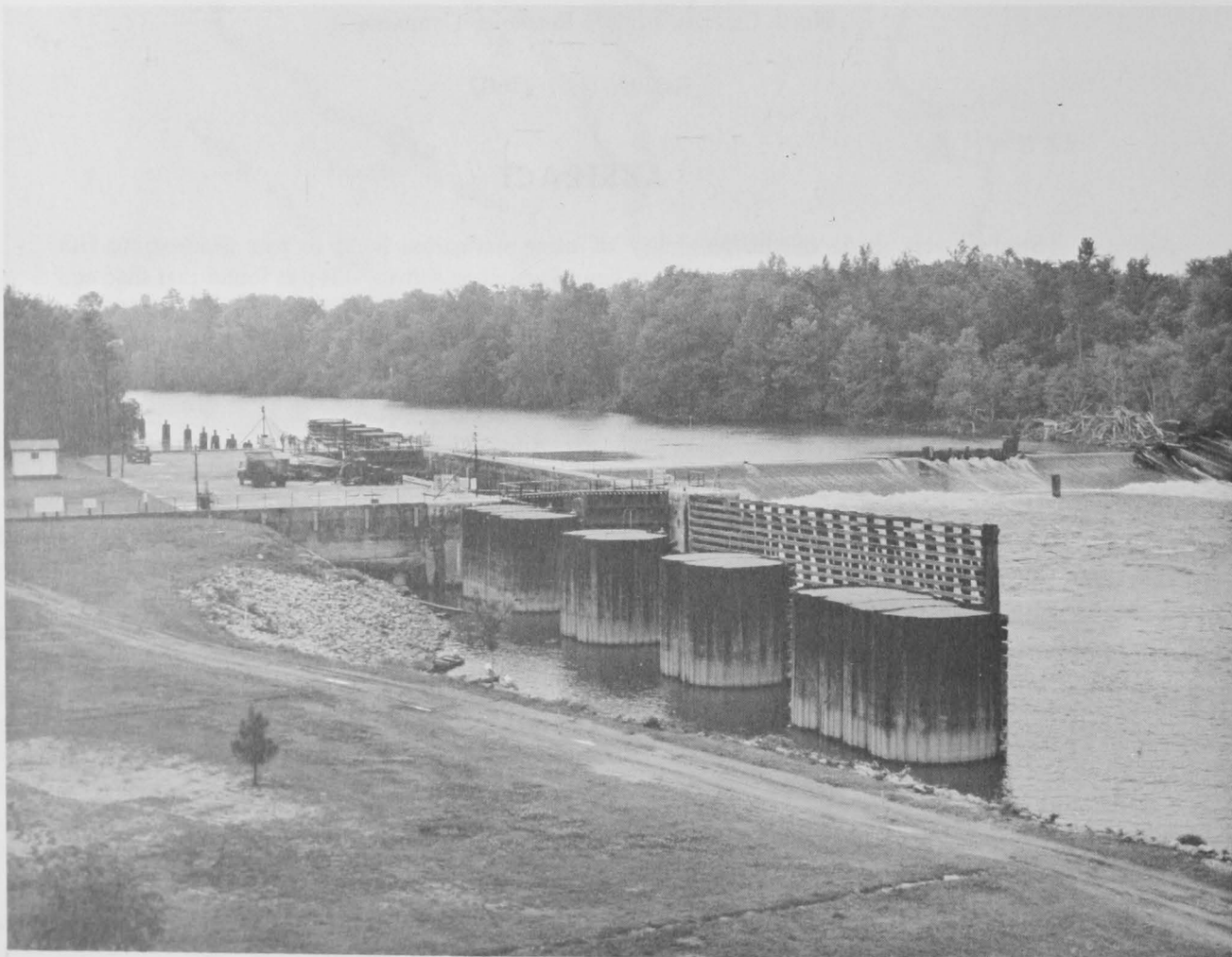
Figure 2.—Lock and Dam 1, Cape Fear River, N. C.
