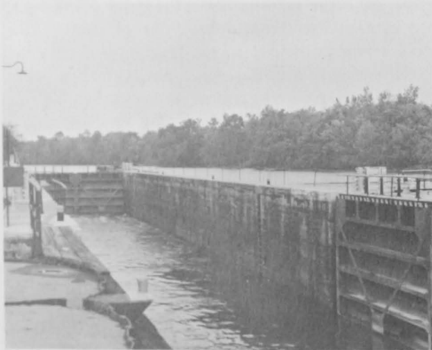
Figure 4.—Navigation lock in position to attract fish from the river below the dam.
