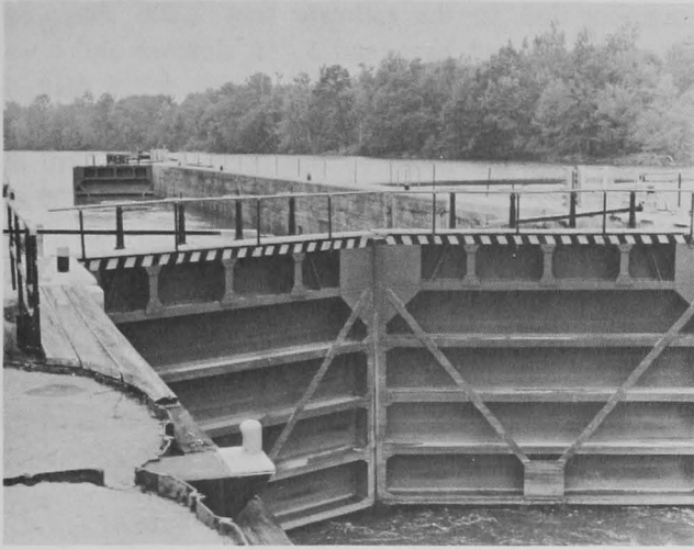
Figure 7.—Navigation lock ready for release of fish from the lock chamber to the river above the dam.
