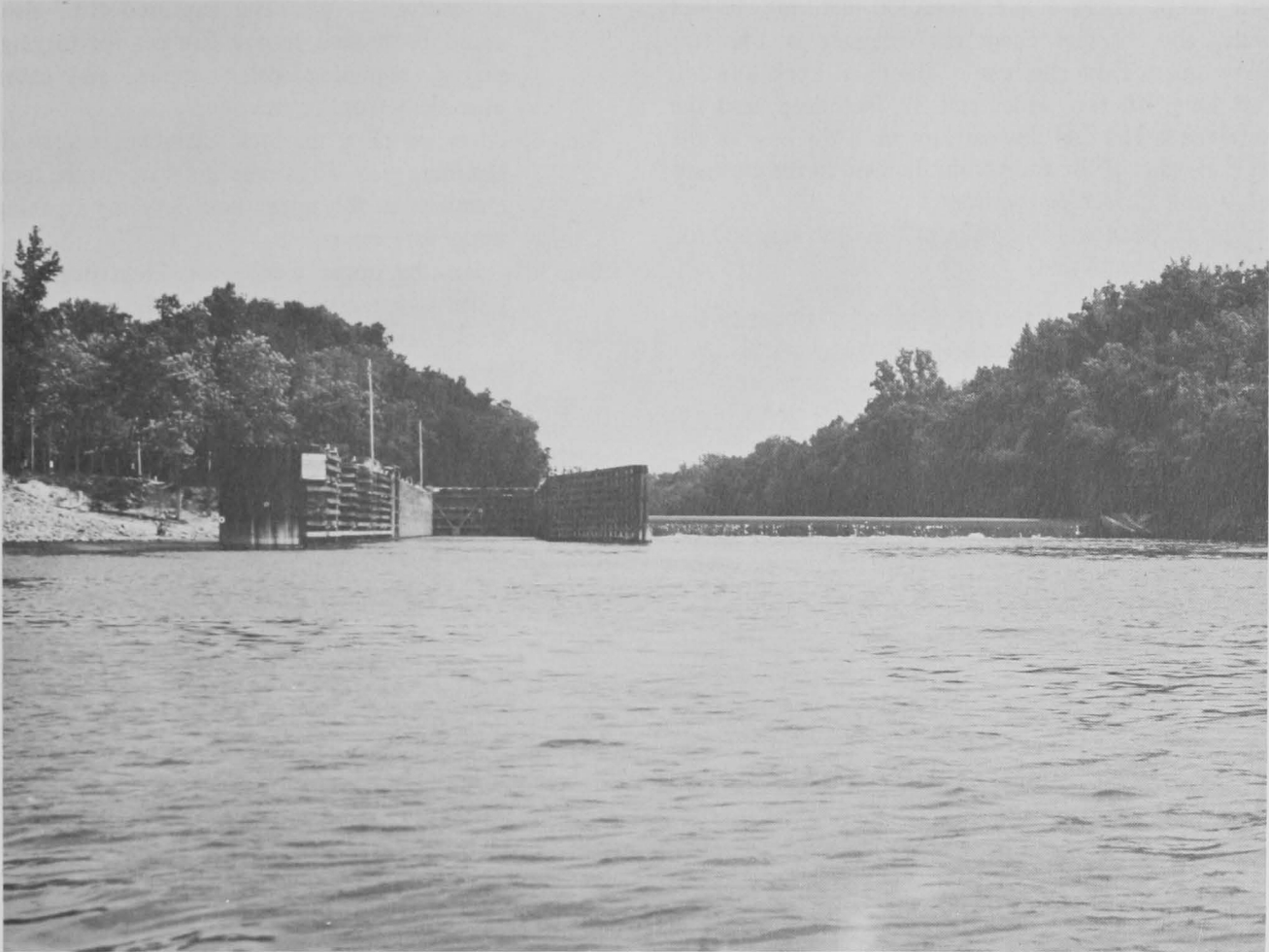
Figure 3.—Lock and Dam 3, Cape Fear River, N. C.
