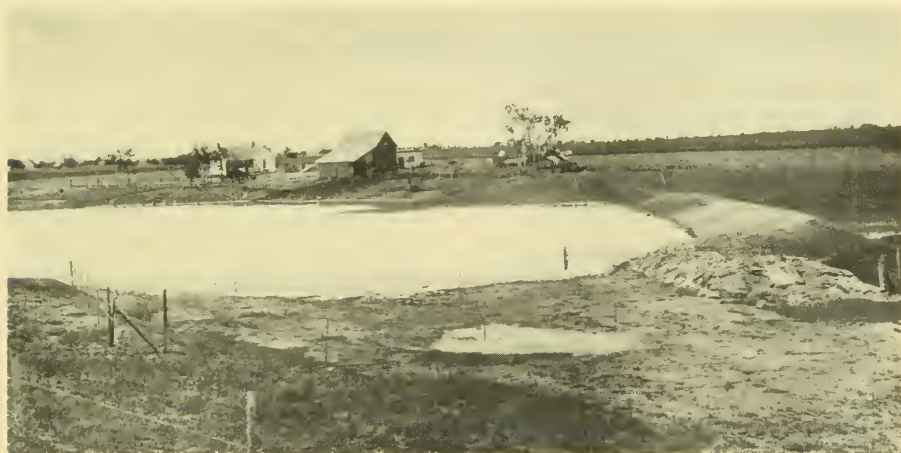
FIGURE 3.—Pond located in a natural gully, using runoff as a source of water. (Photograph courtesy of the U. S. Department of Agriculture.)
