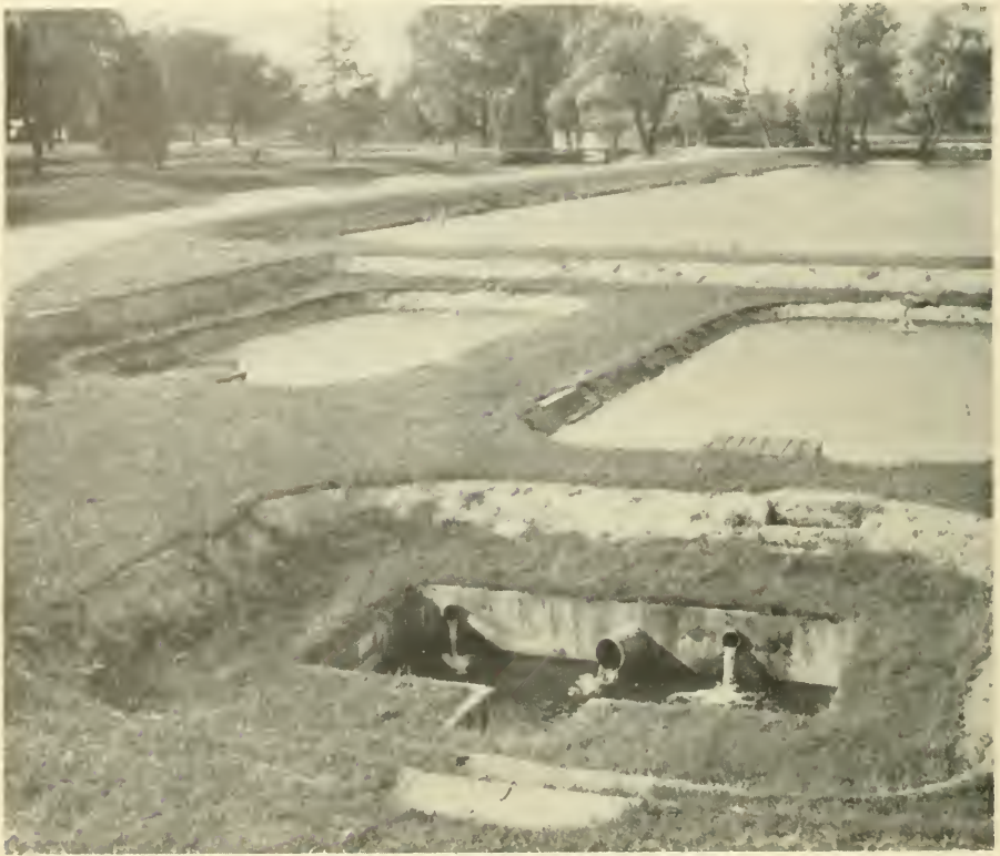
FIGURE 9.—Catch basin constructed outside the pond.
