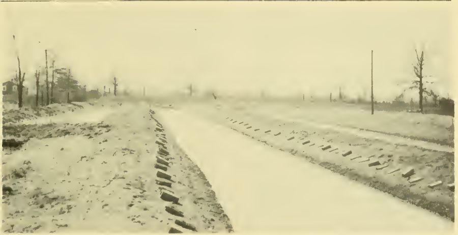
FIGURE 40.—Four-inch tile used for spawning devices. (Photograph courtesy of the Ohio Department of Conservation and Natural Resources.)
