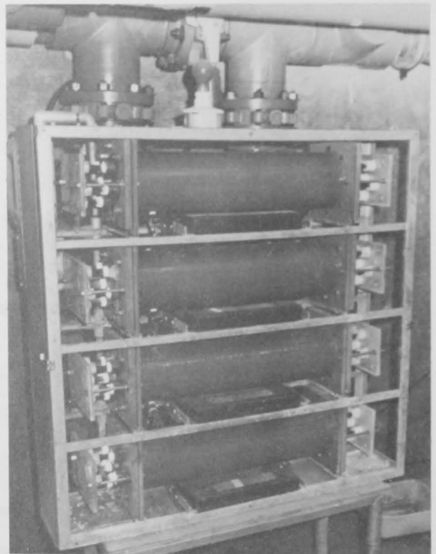
Figure 10. Ultraviolet light sea-water sterilizing unit.
