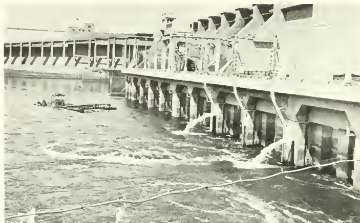
FIGURE 37.—Fish released into turbines at Ice Harbor Dam were collected below the dam. Comparisons were made of the survivals of fish that had passed through turbines and fish that had bypassed the turbines. The hose in the foreground carried the fish that were bypassed.
