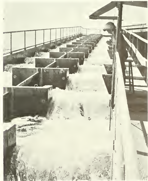
FIGURE 23.—Chinook salmon ascending the fish ladder at Ice Harbor Dam, Snake River.
