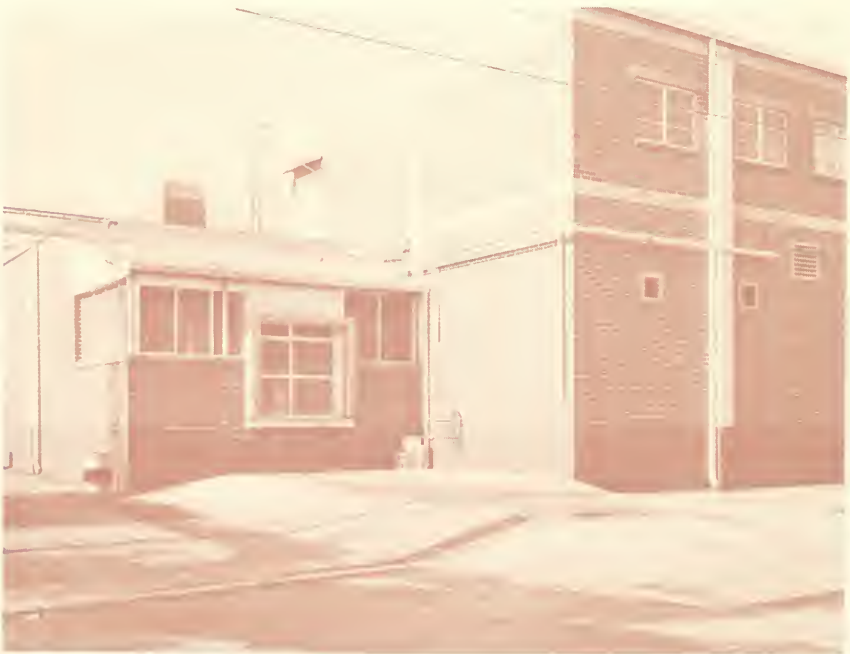
Figure 1.--Modern plant building.
