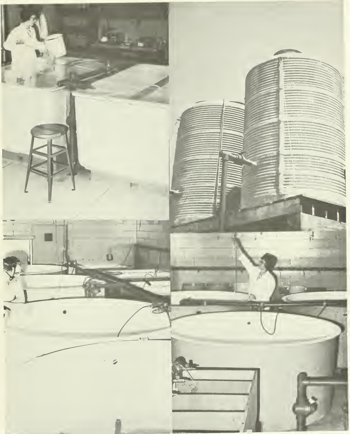
Figure 9.--Salt-water facilities, showing large fiberglass storage tanks (upper right-hand corner) and three sizes of fiberglass tanks inside of laboratory. As far as we can determine, this is the first use of large fiberglass tanks as storage tanks for sea water. Lower right-hand picture shows fiberglass-covered wooden table. Salt-water system consists of a dual set of PVC (polyvinyl chloride) pipes from storage tanks to inside of laboratory. The dual pipe system is alternated weekly--one system is used for salt water while the other system is held as a standby with fresh water for killing organisms that foul the pipes.
