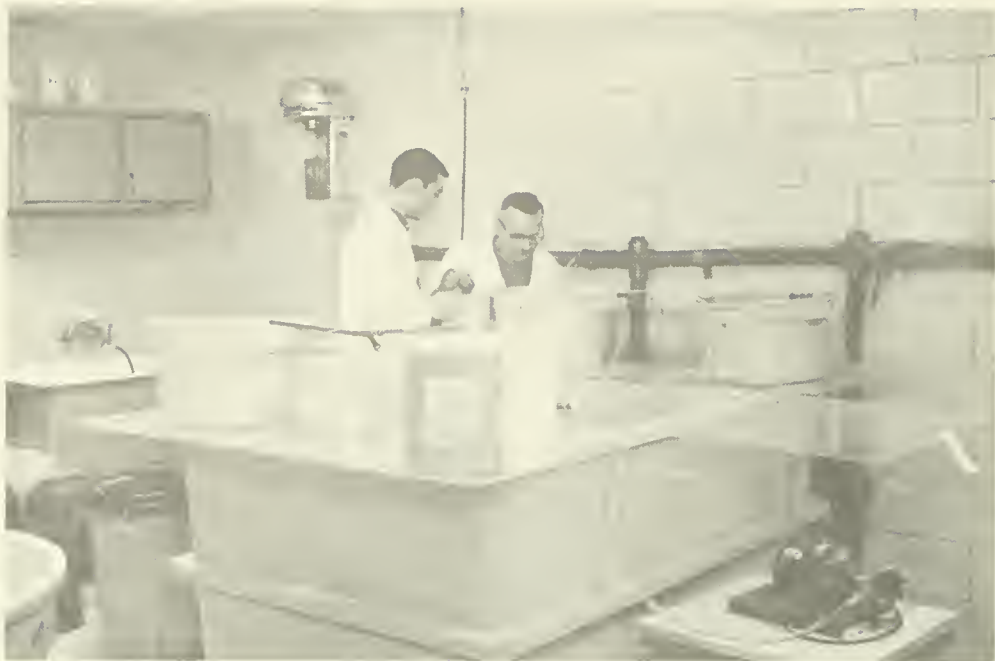
Figure 5.--The effect of environmental factors, such as temperature and salinity, on the accumulation of radioactivity by invertebrates is studied under controlled conditions in the laboratory. Investigators remove organisms from the experimental environment, analyze the live organisms for radioactivity content, then return them to the aquaria. The effect of temperature and salinity on the accumulation of the radioactivity by the organisms is evaluated by statistical analysis of the data.
