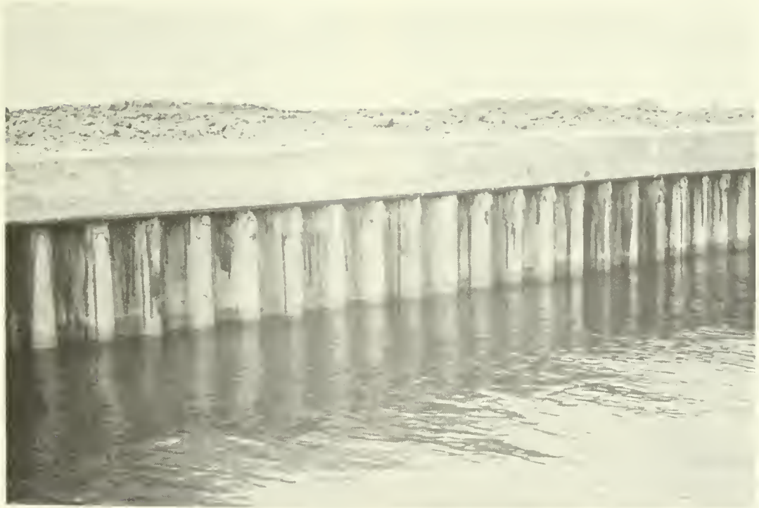
Figure 16.--A former nursery area on west Galveston Island has been developed for housing by bulk-heading the natural shoreline and raising marsh elevation with fill from hydraulic dredging.
