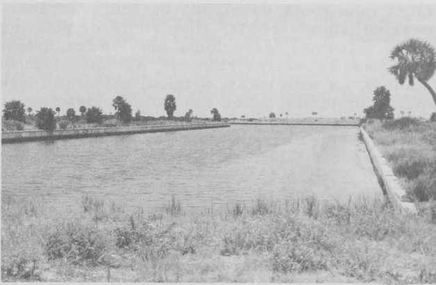
Figure 14.--A typical finger-fill canal in Boca Ciega Bay.
