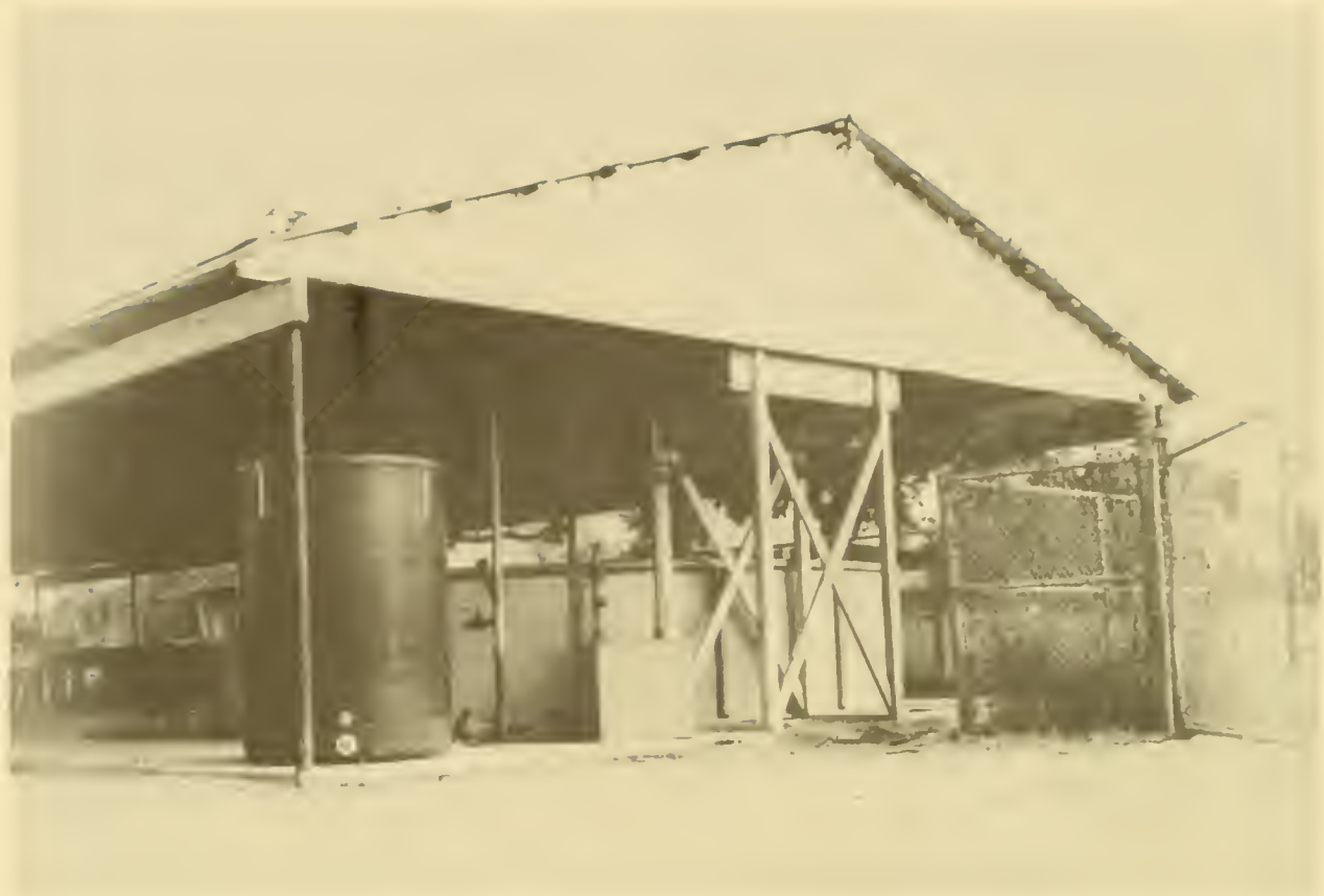
Figure 13.--Partially completed shed holding 7,600-gallon experimental pool.
