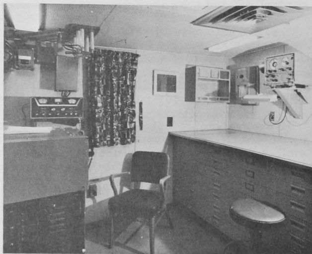
Figure 8.--Radio and chart room showing location of communication and navigational equipment.
